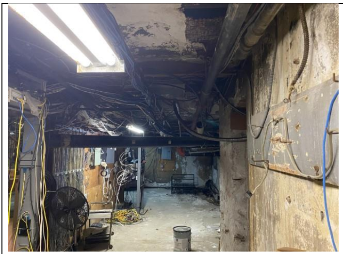
45. Building D basement and foundation.
