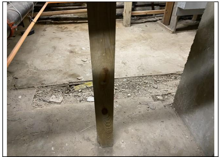
14. Typical structural wood post in the apartment buildings.
