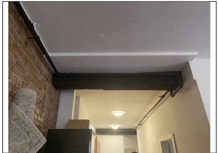
16. Typical exposed heavy timber girder beam in an apartment with acceptable shrinkage cracking.
