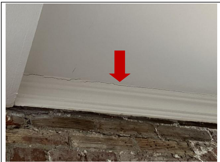
29. Hairline crack visible in apartment ceiling finish.
