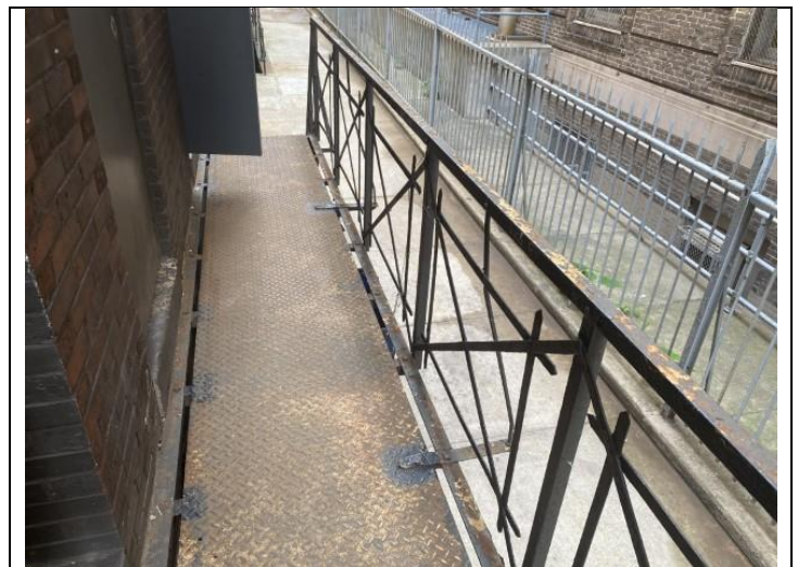
10. Typical cantilevered party-wall egress balcony.
