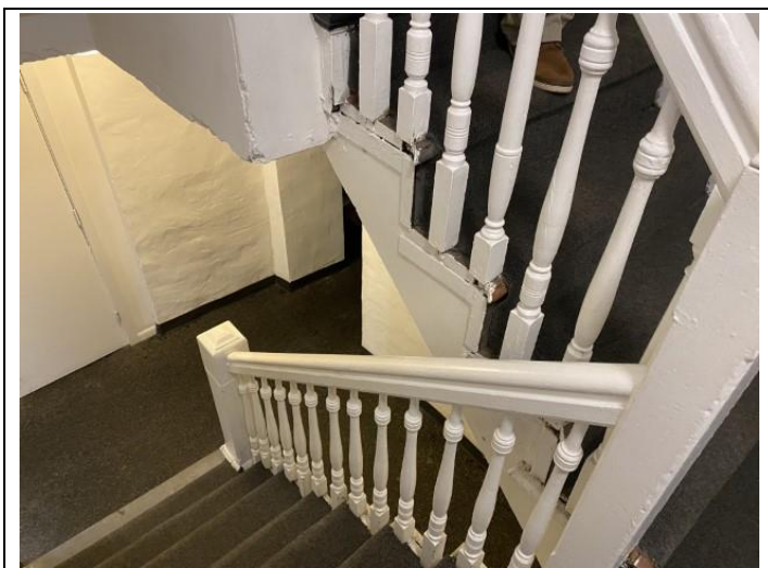
11. Typical interior staircase to basement framing.
