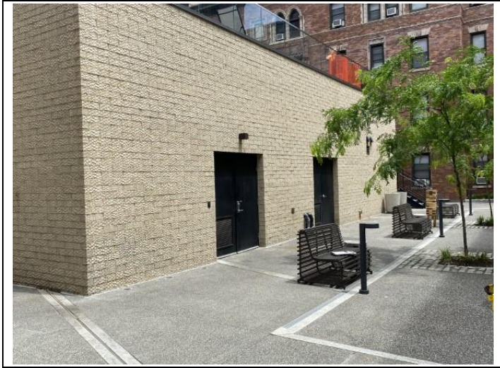
19. Partial south elevation of the Amenity Building.
