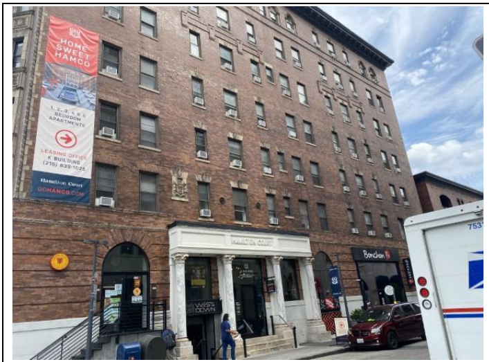
3. Partial west elevation of Buildings K and J from South 39th Street.
