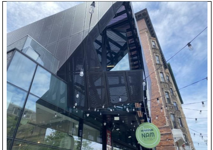
18. Amenity Building curtainwall and aluminum veil as seen from Chestnut Street.
