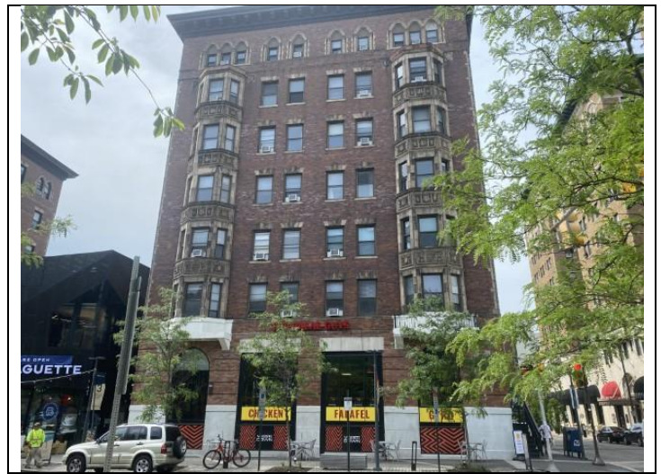
2. Full south elevation of Building K from Chestnut Street.
