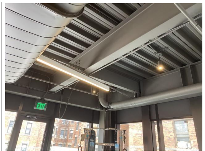
23. Typical exposed wide-flange beam and floor decking in the Amenity Building.
