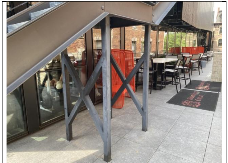
22. Amenity Building steel exterior staircase framing.
