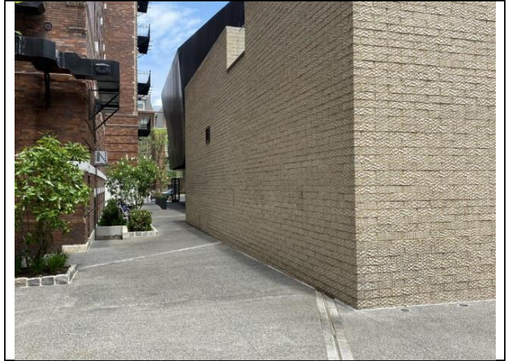
20. Partial west elevation of the Amenity Building.
