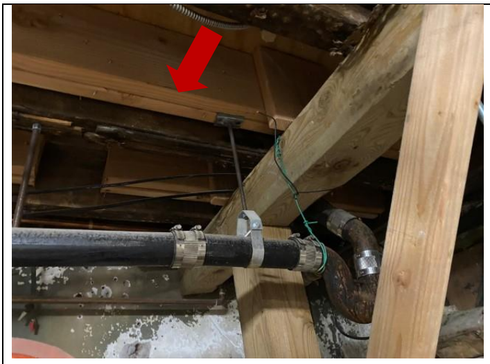
43. Sistered wood floor joists.
