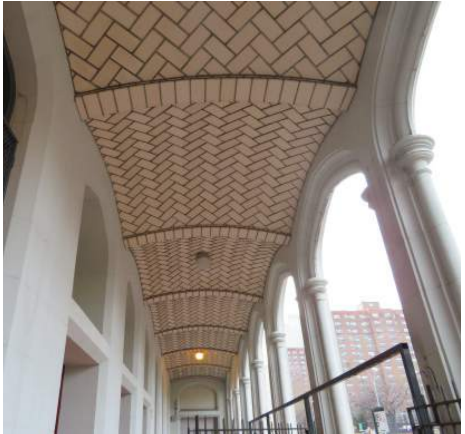
Top left: tiled ceiling before restoration. Bottom left and center: ceiling during construction. Top right and bottom right: restored Guastavino tile ceiling.
