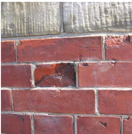
Top left: Deteriorated brick before. Top right: Matching brick in kind. Bottom left: Brick spalling. Bottom center: Brick on tower during replacement. Bottom right: Brick after.
