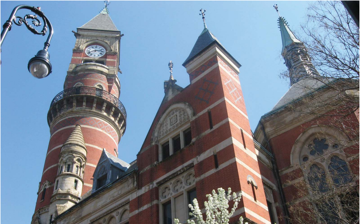
425 Avenue of the Americas prior to restoration
