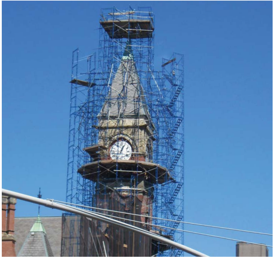
Top left: Tower cap during restoration. Top right: Scaffolding allowing work to be done on tower cap and finial. Bottom left and center: Newly fabricated copper finial on tower cap during restoration. Bottom left: Interior of tower cap.
