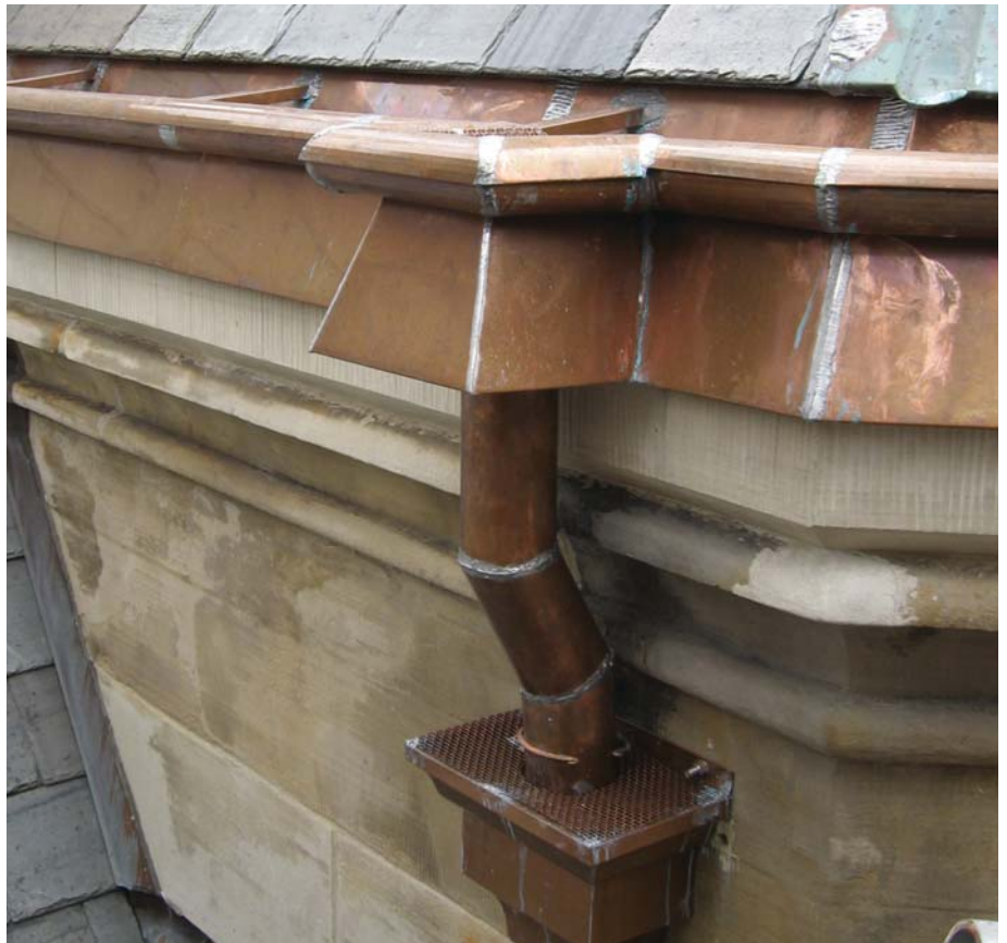
Top left and bottom left: Gutters and leaders before. Bottom center and right: New copper gutters during installation. Top right: Gutter and leader after.
