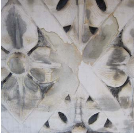
Top left: Deteriorated stone before restoration. Bottom left: Stone ornament after re-carving. Top right: Re-carving stone in place. Bottom center: Deteriorated stone before. Bottom right: Newly carved stone ornament replaces highly eroded original carving.
