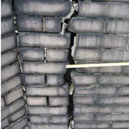
Top, left: Brick deterioration before restoration. Top, right: Brick after restoration. Bottom, left: angled brick used before to tie courses together. Bottom center: Brick displacement at spandrel level. Bottom right: matching new brick to original.
