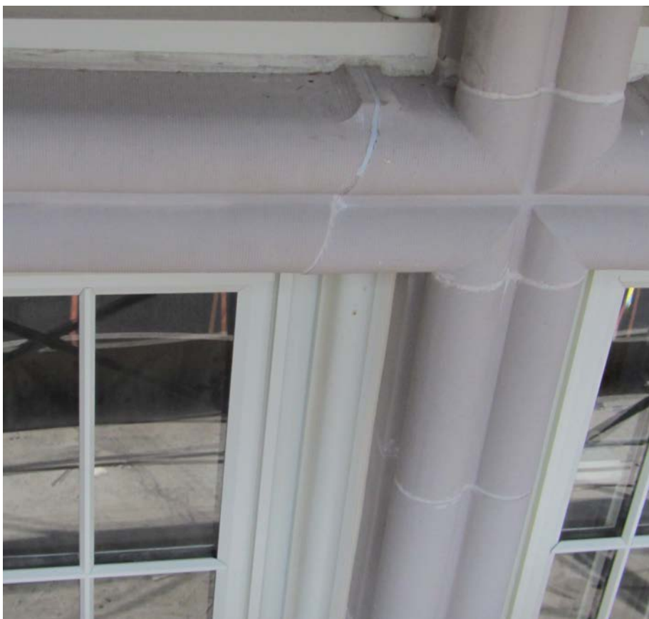
Top, left; bottom, left; bottom, center: Deteriorated terra cotta. Bottom, left: New terra cotta installed. Top, right: New terra cotta after.
