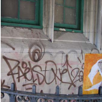
Top, left: Graffiti covered limestone. Top, right: Limestone cleaned. Bottom, left: Ornamental limestone before. Bottom, center: Ornamental limestone after. Bottom, right: Limestone cleaning in progress.
