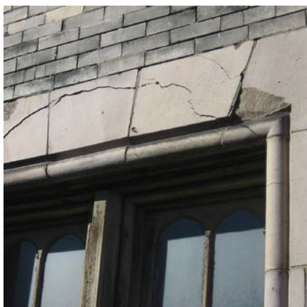
Top, left; bottom, left; bottom, center: Deteriorated terra cotta. Bottom, left: New terra cotta installed. Top, right: New terra cotta after.
