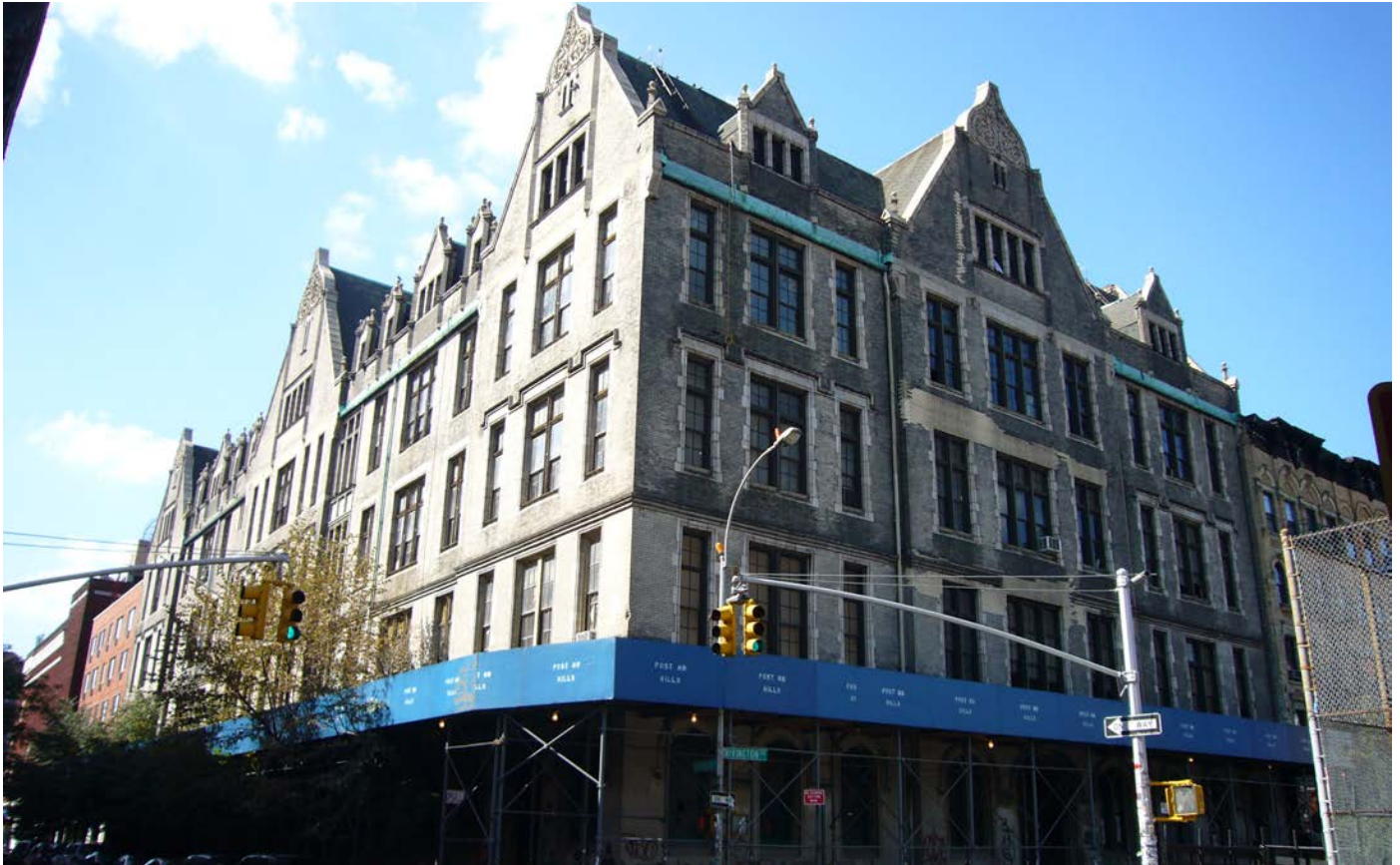
107 Suffolk Street prior to restoration
