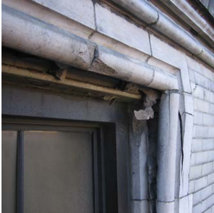
Top, left; bottom, left: Terra cotta before. Bottom, center: Spalling and displaced terra cotta bracket. Bottom, left: Terra cotta bracket after. Top, right: Terra cotta after.
