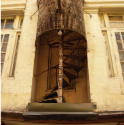
Top, left and right; bottom, left: Spiral stair and lattice cage before restoration. Bottom, center and right: Spiral stair and lattice cage after restoration.
