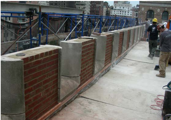
Parapets during reconstruction.
