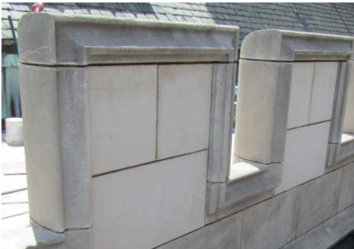
Parapets during reconstruction.
