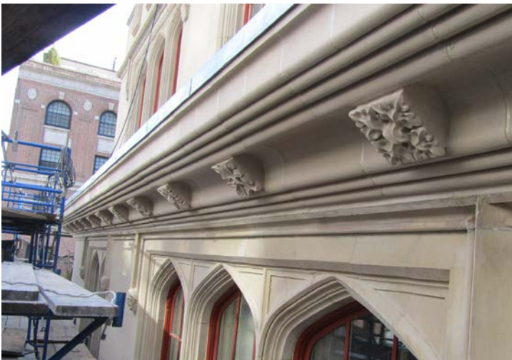
Completed cornice with GFRP replicating original terra cotta cornice details.
