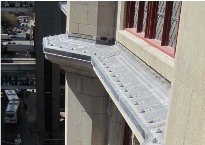
Completed roof over new cornice.
