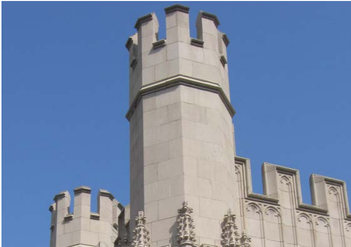
Reconstructed and cleaned turrets.
