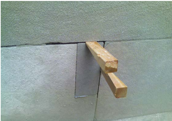
Dutchman repair to limestone. Patching was done in more ornate areas.
