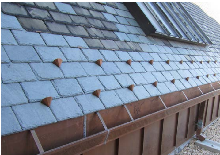
Slate roof after restoration. Original building fabric was retained where possible.
