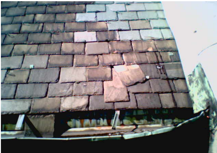
Slate roof and copper gutter before restoration.
